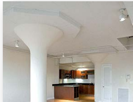
System 2: flat slab with drop panel
