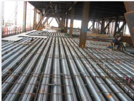
System 1: (existing) beam with metal decking
