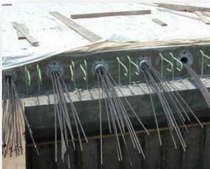
System 3: Post Tension conc. slab
